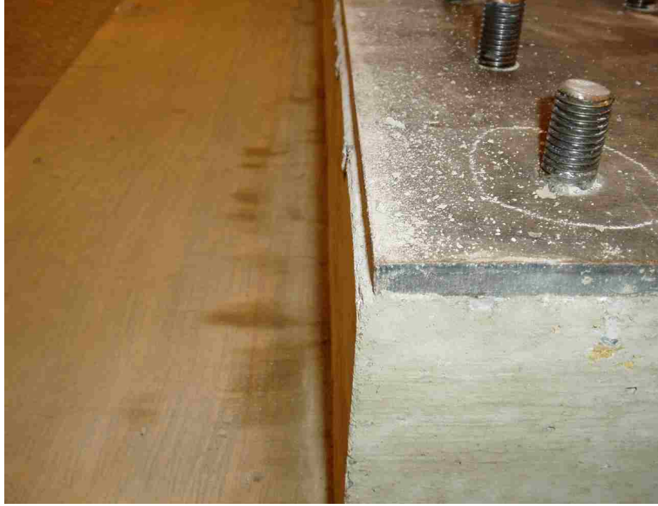
Figure 4-10 - Excess Concrete to be Removed after Curing was Complete
