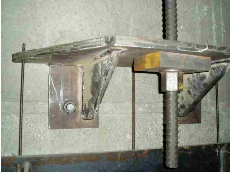
Figure 4-15 - Lifting Attachment
