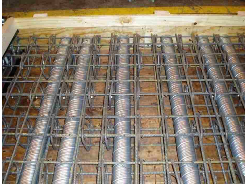
Figure 4-6 - Rebar Cage Detail
