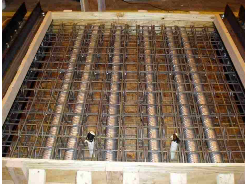
Figure 4-1 - Formwork with Rebar Cage and Post-Tensioning Steel Ducts in Place
