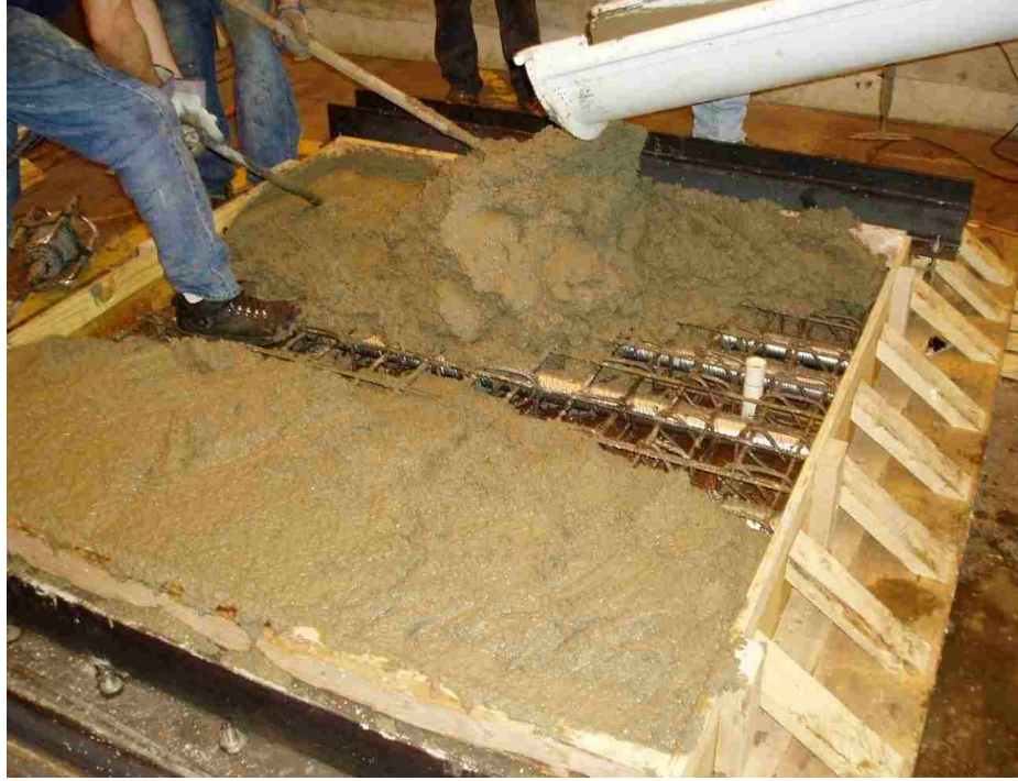
Figure 4-8 - Pouring the Panel
