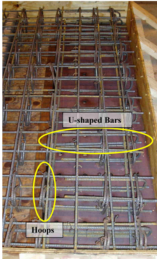
Figure 3-8 - Detail of the Rebar Cage in the Plate-confined Region
